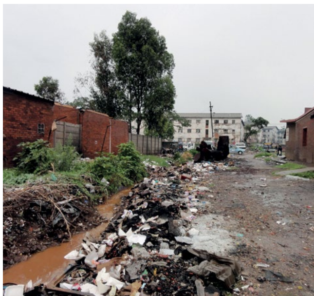
Blocked drains from solid waste Mbare, Harare. P Feiereisen, 2011 under CC
